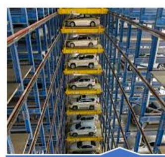
Robotic Parking System
