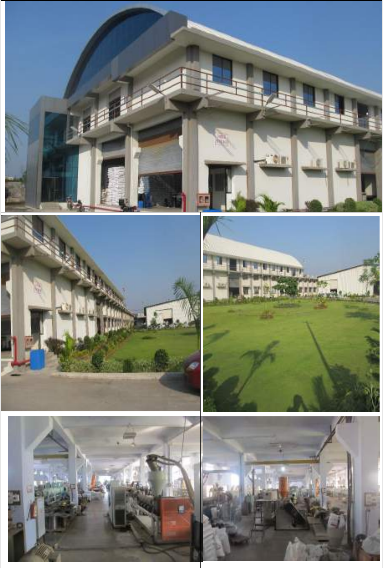
Photos of our Manufacturing Facility-1
